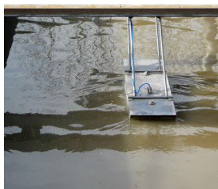
Patented float solution for detection of flow and sedimentation.
